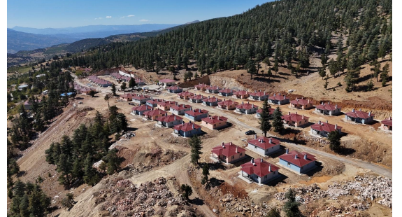
OSMANIYE STAGE 4 RURAL POST-EARTHQUAKE HOUSING, 2025
