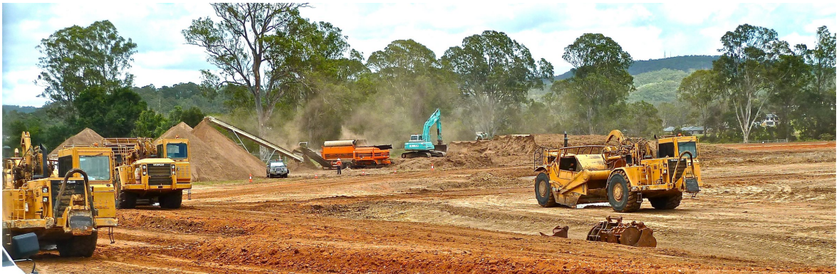
SITE PREPARATION AND EARTHWORKS
